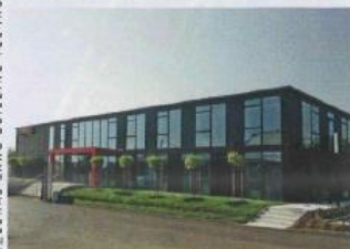
C. LUKAS LANG, BUILDING TECHNOLOGIES GMBH
